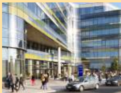
Figure 67. Commercial building. Source: ADT, n.d.
